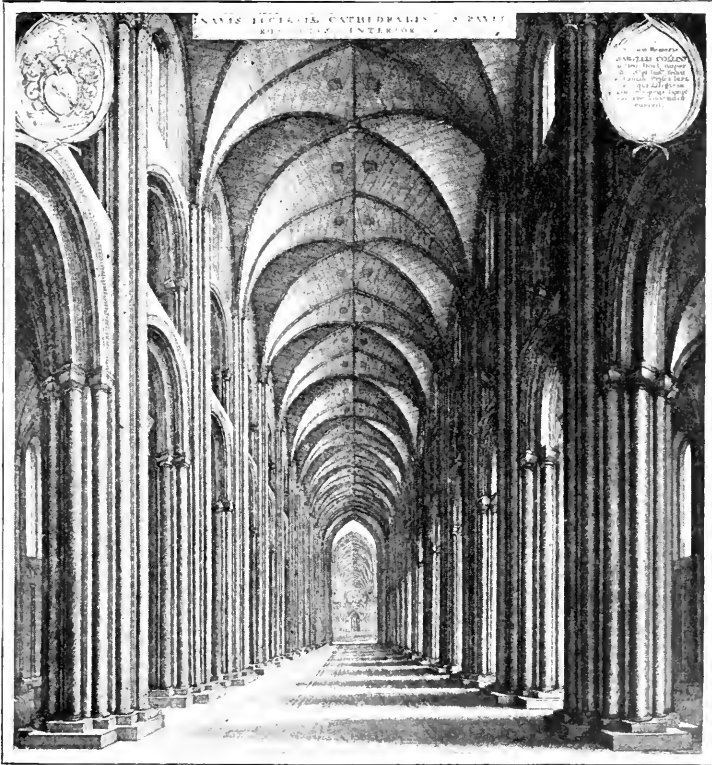
NAVE OF OLD ST. PAUL'S.
